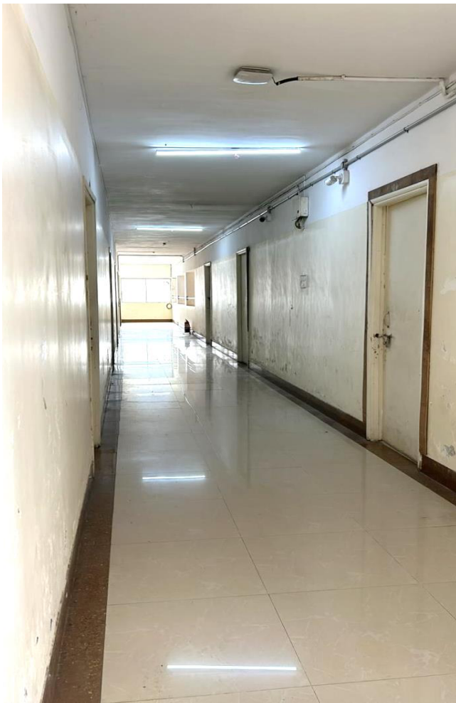
Back block of hostel for senior batch students under CCTV
